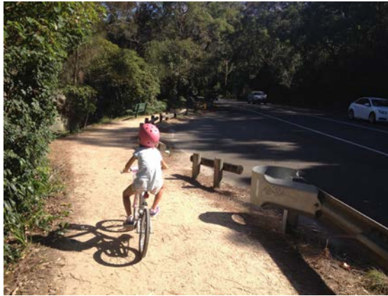
Figure 2: Narrow exiting trail with unprotected openings to 70km/h roadway
