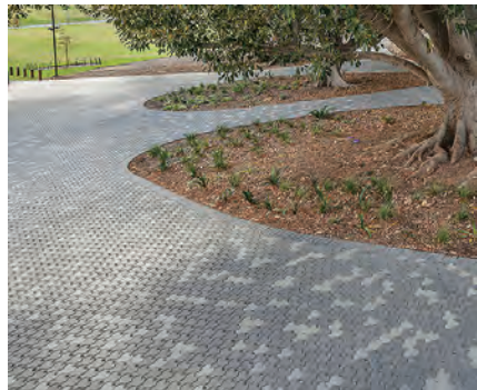
Car Park Permeable paving for parking bays to reduce run-off & enhance tree growing conditions
