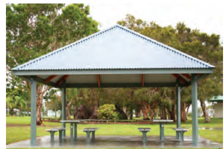
Colorbond roofing (Colour: Windspray) with hardwood timber framing
