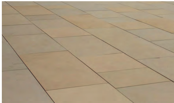
Sawn sandstone feature paving at entry & central meeting point
