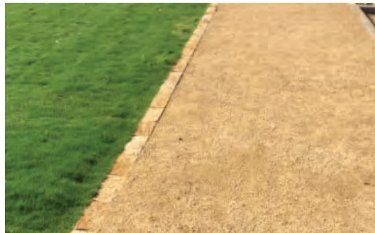
Decorative gravel surfacing (stabilised) with sawn sandstone edging to main promenade
