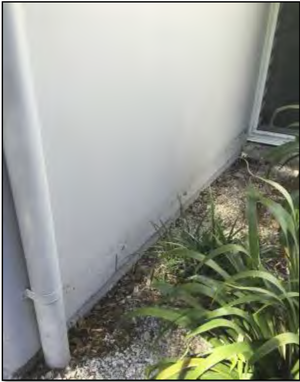
Plate 7 Flood debris line on an external wall at a residence in Howell Close following the November 2015 flood
