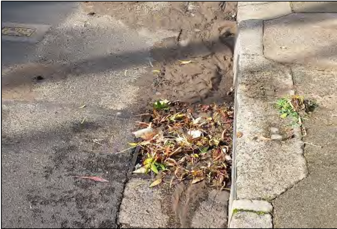
Plate 12 Typical blockage of a stormwater pit
