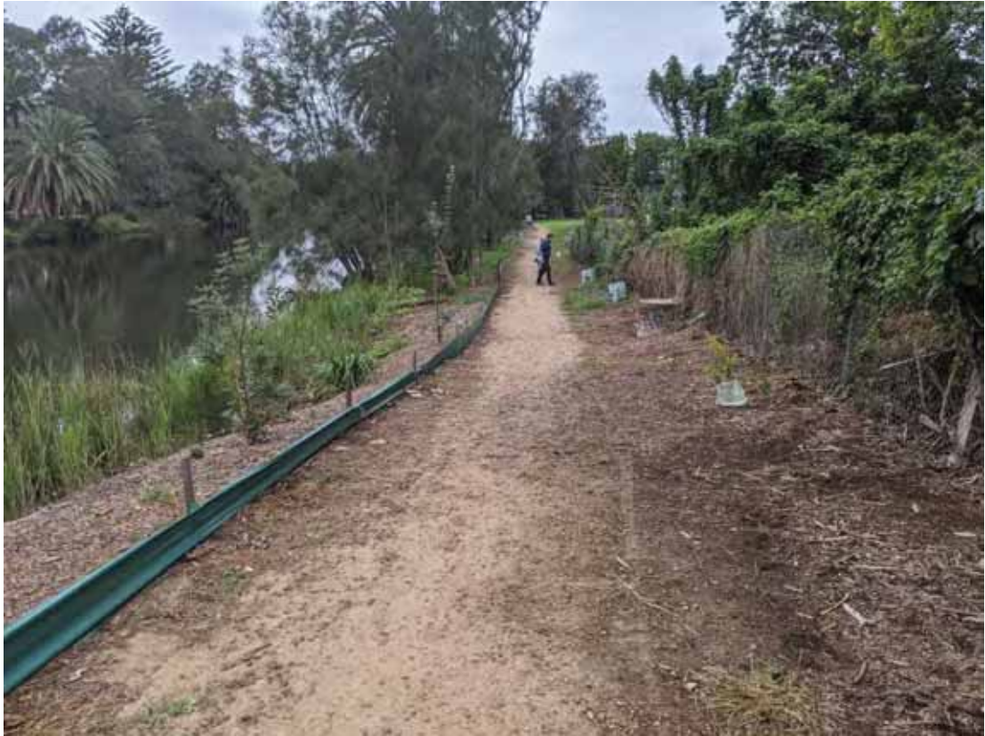
Photograph 3 Facing south along the eastern footpath, showing the sediment fences installed on the eastern site boundary
