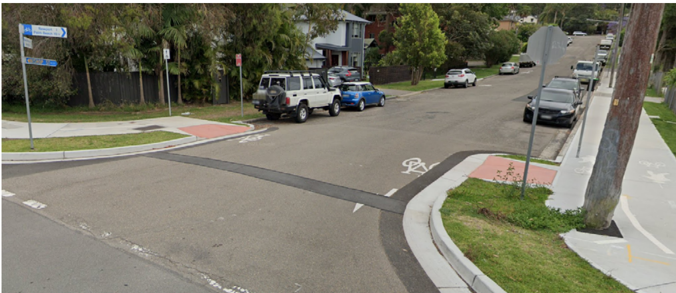
Safer Crossing Treatment Example Bent out crossing with kerb extensions (Bishop Street, Newport)
