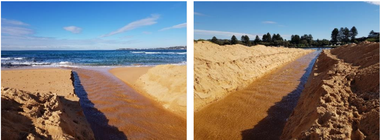
Figure 2-15: Mechanical opening of the lagoon entrance (4 June 2021)
