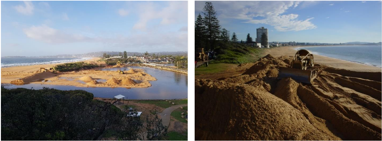
Figure 2-16: Excavators removing the entrance shoals (left), Unloading and regrading of sand for beach replenishment (right)
