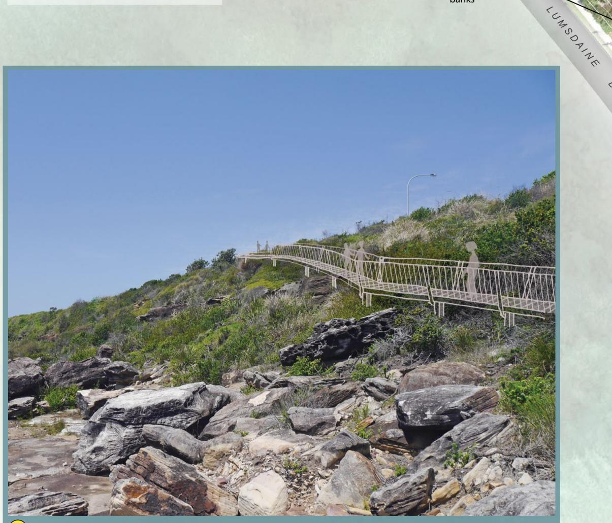
SKETCH CONCEPT OF ELEVATED BOARDWALK THROUGH VEGETATION Sensitvely designed elevated boardwalk is situated above and clear of the existing native vegetation supported on posts attached to the rock below, resulting in minimal impact to indigenous vegetation and the visual character of the area. The proposed alignment will traverse at a gentle gradient through an area of younger vegetation to avoid damaging mature native species in nearby steep coastal banks.
