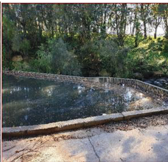
Photo 7: GPT trash rack (looking downstream)
