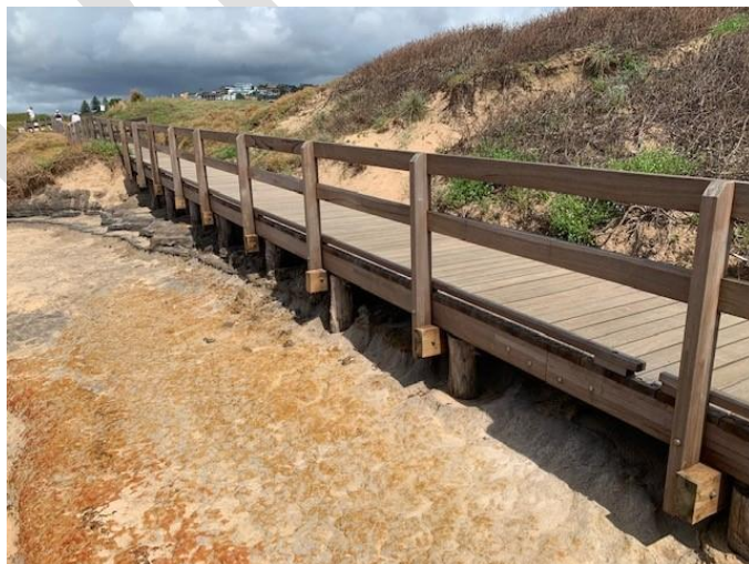
Photograph 6: Scouring of sand adjacent to boardwalk, exposing reddish clay material
