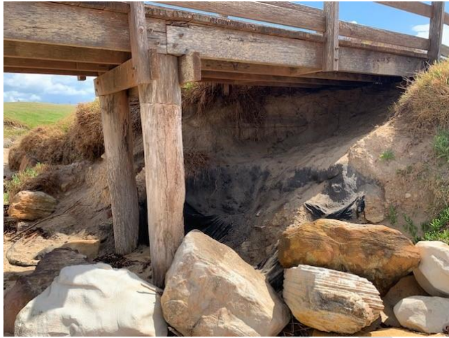
Photograph 4: Rock armoring at northern end of bridge
