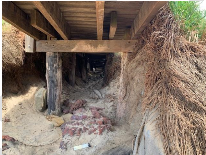
Photograph 5: Scouring of sand dune below southern end of bridge approach
