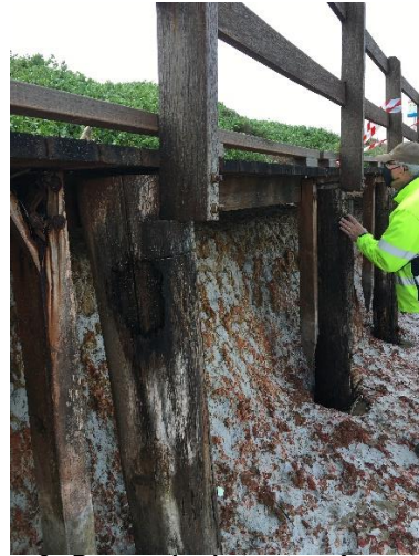
Figure 2 - Damaged substructure August 2021
